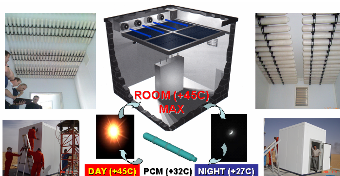
Figure 4.3.5- Passive electronic shelter cooling applications.
