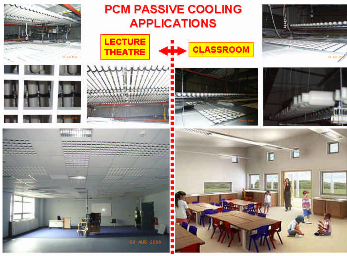
Figure 4.3.4. Passive cooling UK school application examples.
