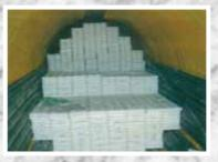
FlatICE containers can only be stacked up to a height of 2.6 m (8 ½ ft) and therefore the height of the tank is restricted to around 3m (10 ft) and the foot print of the tank can be adjusted around this limit.
