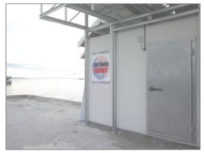
It is energized by a 6.4 kWp solar array through a 3-phase inverter system, backed up by a relatively small 10 kWh VRLA battery bank.
