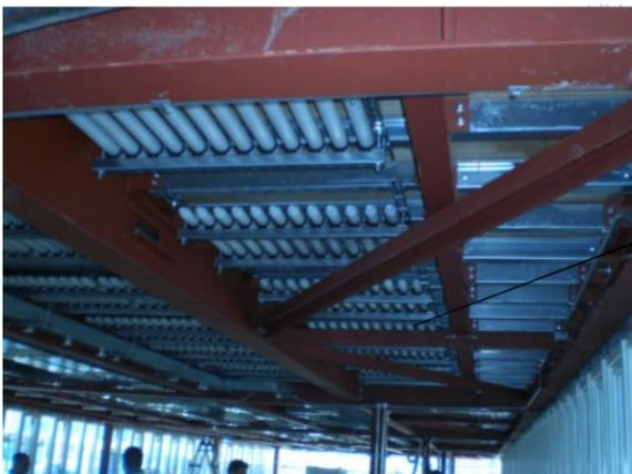
Over night, PCM tubes fitted within the ceiling area freeze naturally by the surrounding cooler night ambient and later this stored energy in the form of latent heat is released back to the system during daytime to absorb the internal heat gains. As the heat tends to rise and using the temperature stratification within the room rising heat melts the tubes and cooler airdrops back to occupied space and the PCM filled tubes acts like a heat sponge and soak up the heat during daytime.
