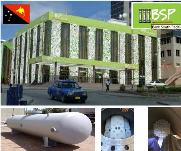
As the cooling load having large peaks it was vital to shift the loads and spread over 24 hours period. To this end 12 m<sup>3</sup> tank containing FlatICE containers filled with S8 (+8C/47F) providing 420 kWh (120 RT-h) TES capacity.
